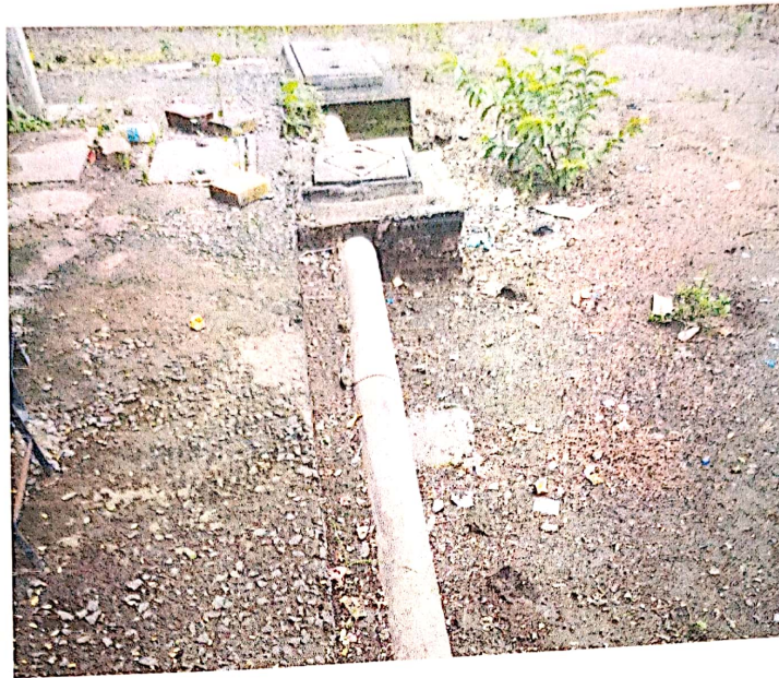
Waste pipe with Chambers
